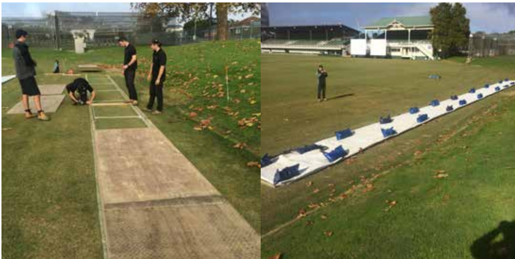
Trial structure being built and covered on June 15 2016
